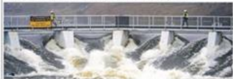
Workers are reinforcing the dam as the river runs high. The dam is part of a $1.4-billion project to build a new dam on the Huron River in Michigan.
